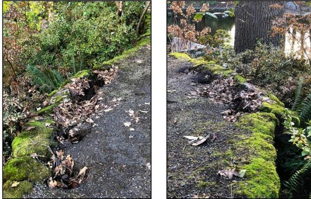
*These photographs show one of the retaining walls beginning to pull away from the upper pathway above the Flowerree Memorial Garden at Crystal Springs. The pathway has been closed until the retaining walls can be rebuilt and the hillside stabilized.*
